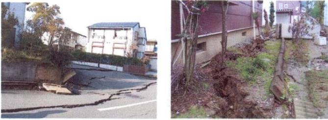
Fig.4 (a) Fractures and faulting near perimeter edge (b) Fractures and faulting of residential land
