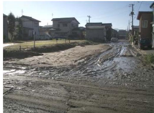
Fig.9 Road buried under sand boil
