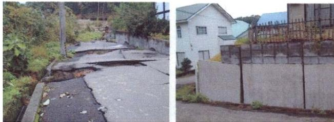
Fig.5 Road collapse caused by landslide
