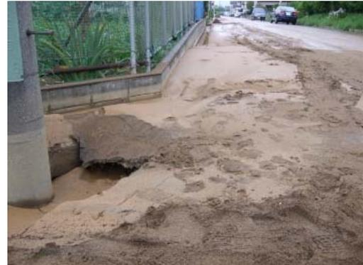
Fig.18 Sand boil caused by liquefaction
