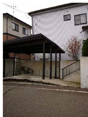
Fig.13 House settlement and upheaval of earth floor
