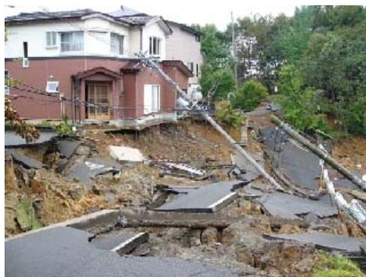
Fig.2 Collapse of buried ravine earthfill
